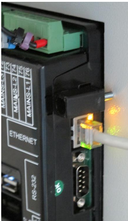
Installation of screw type bracket
