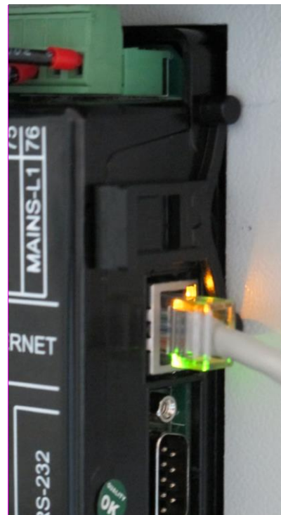
Installation of self-retaining type bracket
